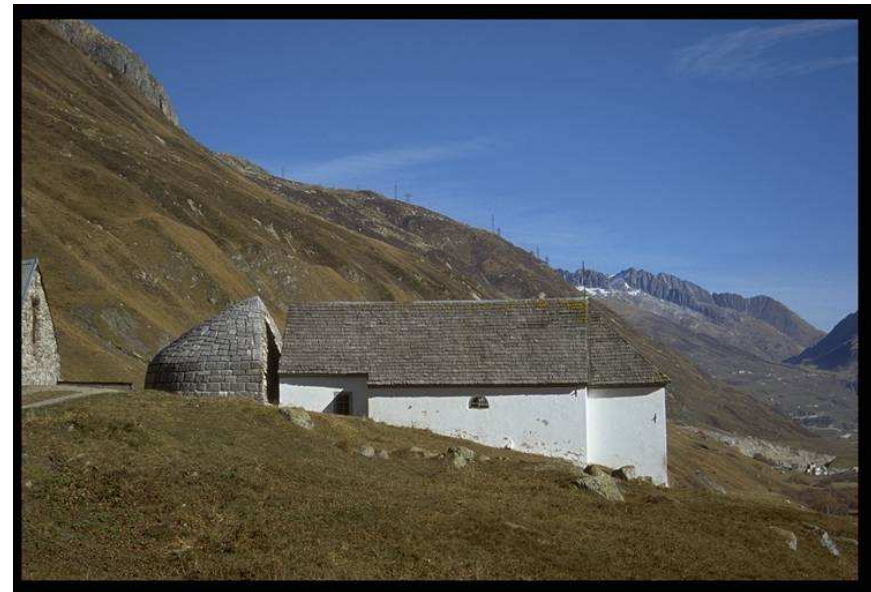
Passive defense structure
