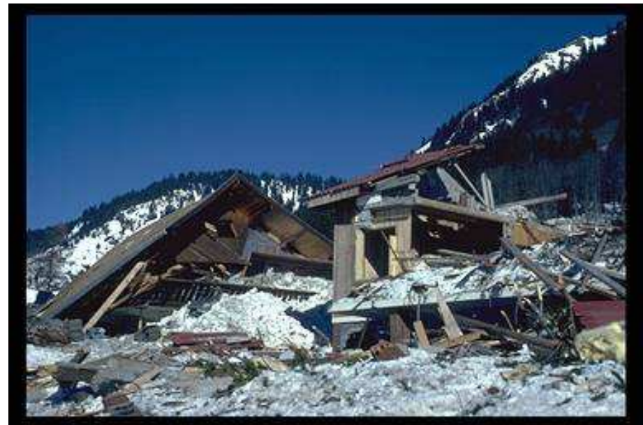
House destroyed by a powder snow avalanche, French Alps
